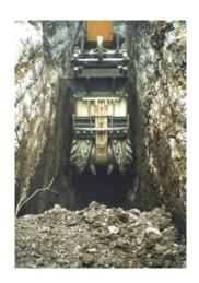
A grinder head can cut through several layers of rock, pavement, concrete and soil.
