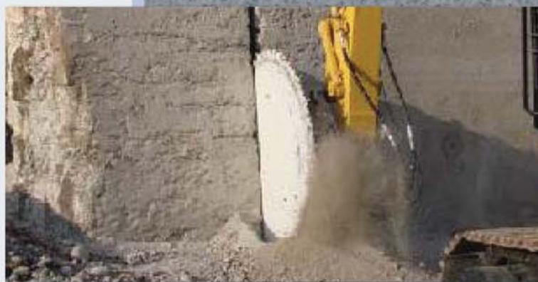
Precision block cuts, trenching, demolition & more
